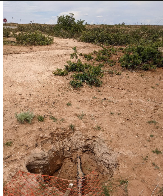
Photograph 4 Date: June 21, 2022 Description: View of remediation excavation
