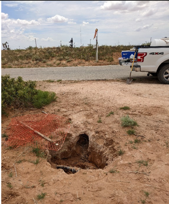
Photograph 3 Date: June 21, 2022 Description: View of remediation excavation
