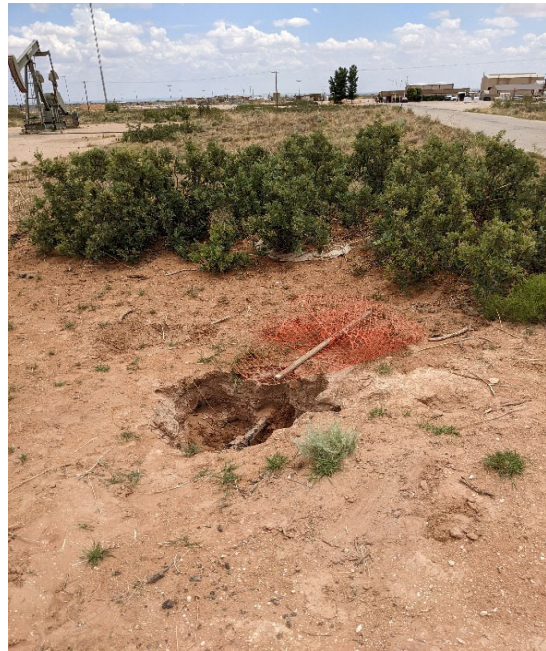
Photograph 2 Date: July 21, 2022 Description: View of the remediation excavation.
