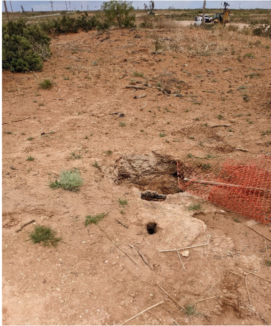
Photograph 1 Date: June 21, 2022 Description: View of remediation excavation
